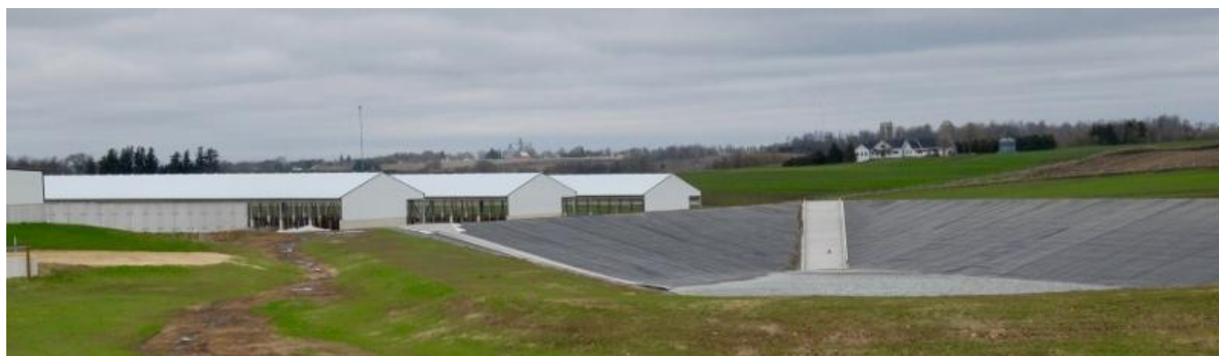
Supreme Beef 4-21-2021 with 38+ million gallon fabric lined lagoon. Photo by Larry Stone
